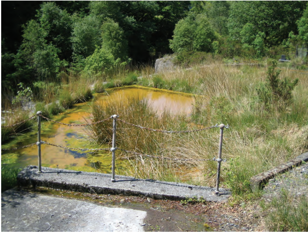
Plate 7.3 A disused limestone filter bed constructed in the 1960s to treat Cwm Rheidol mine discharge (Source: original)
